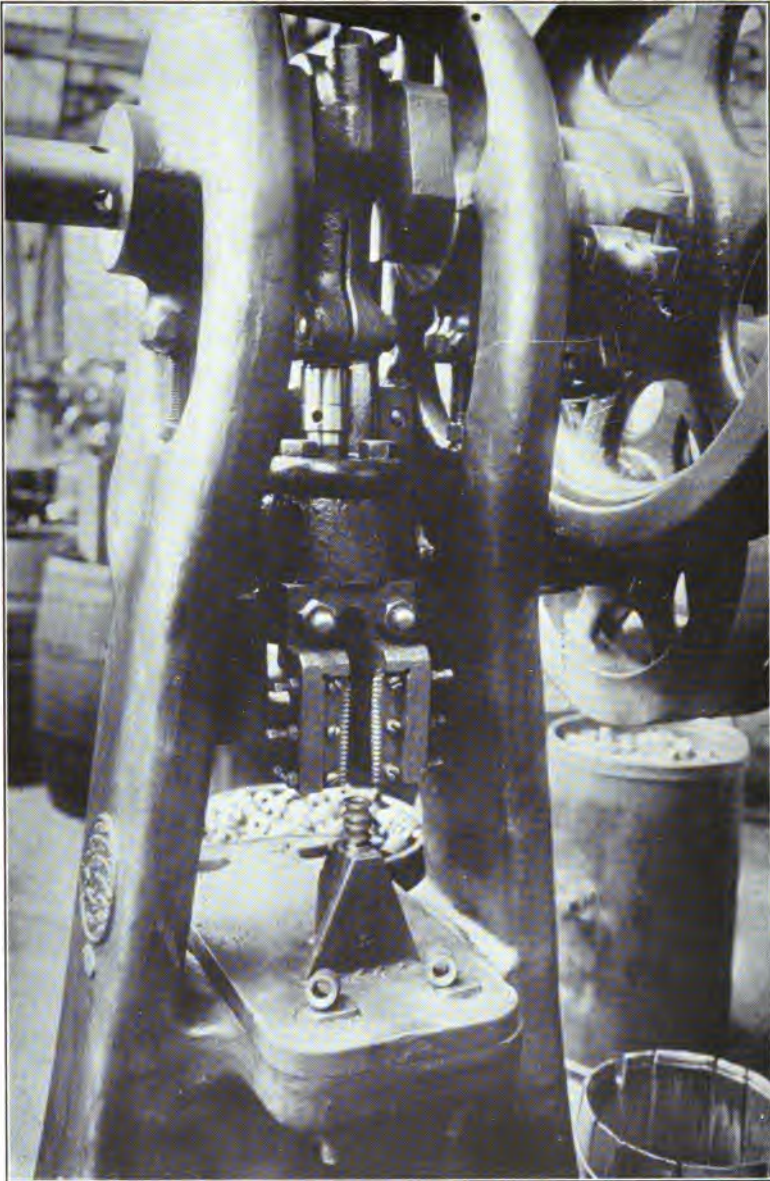
FIG. 82.—External broaches for splitting bearings.
